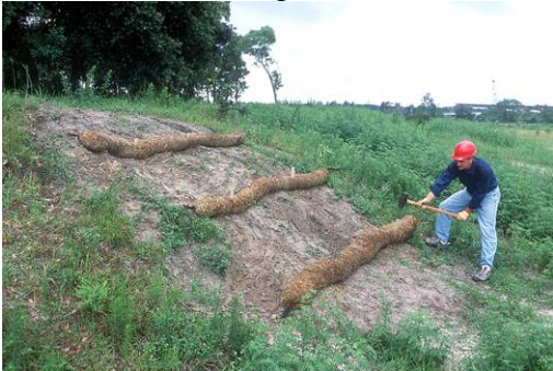
Wheat straw rolls being used to stabilize a slope
